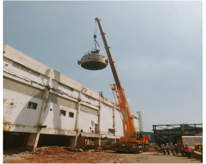
Lifting & Shifting of Tank (weight 15 Tonnes over wall Height 15 Mtr.)
