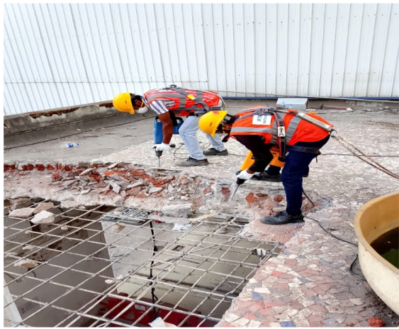
250mm RCC Slab Breaking in progress
