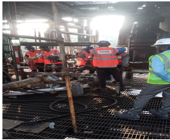
Process pipe removal in progress
