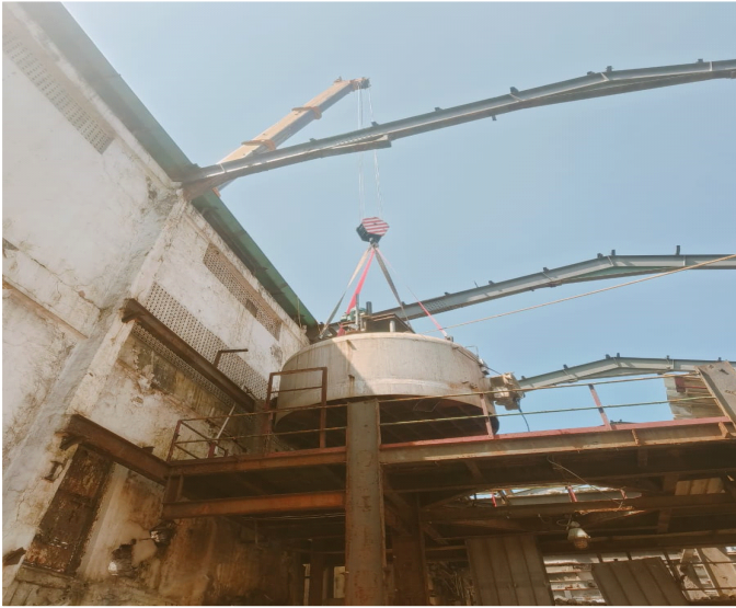
Lifting & Shifting of Tank (weight 15 Tonnes over wall Height 15 Mtr.)
