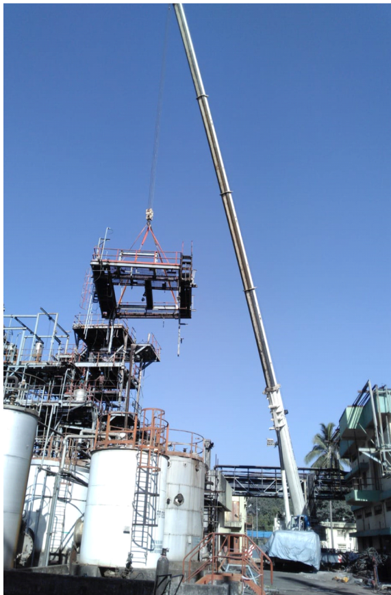
Removal of Structure column & Staircase work in progress
