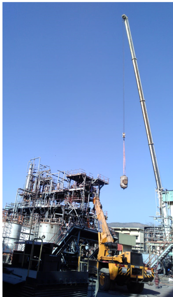
Dismantling of large distillation column work in progress
