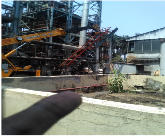
Removal of Structure column & Staircase work in progress
