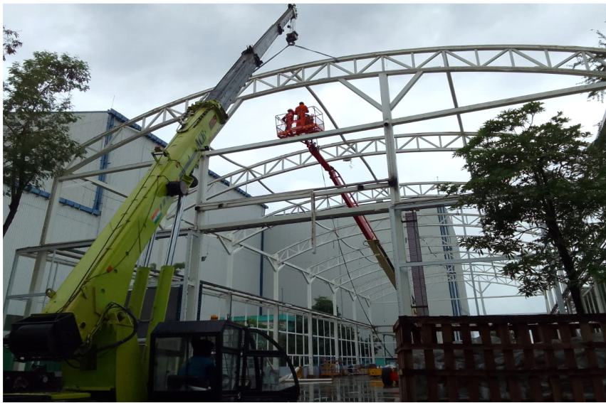
Removal of Tensile cloth & structure
