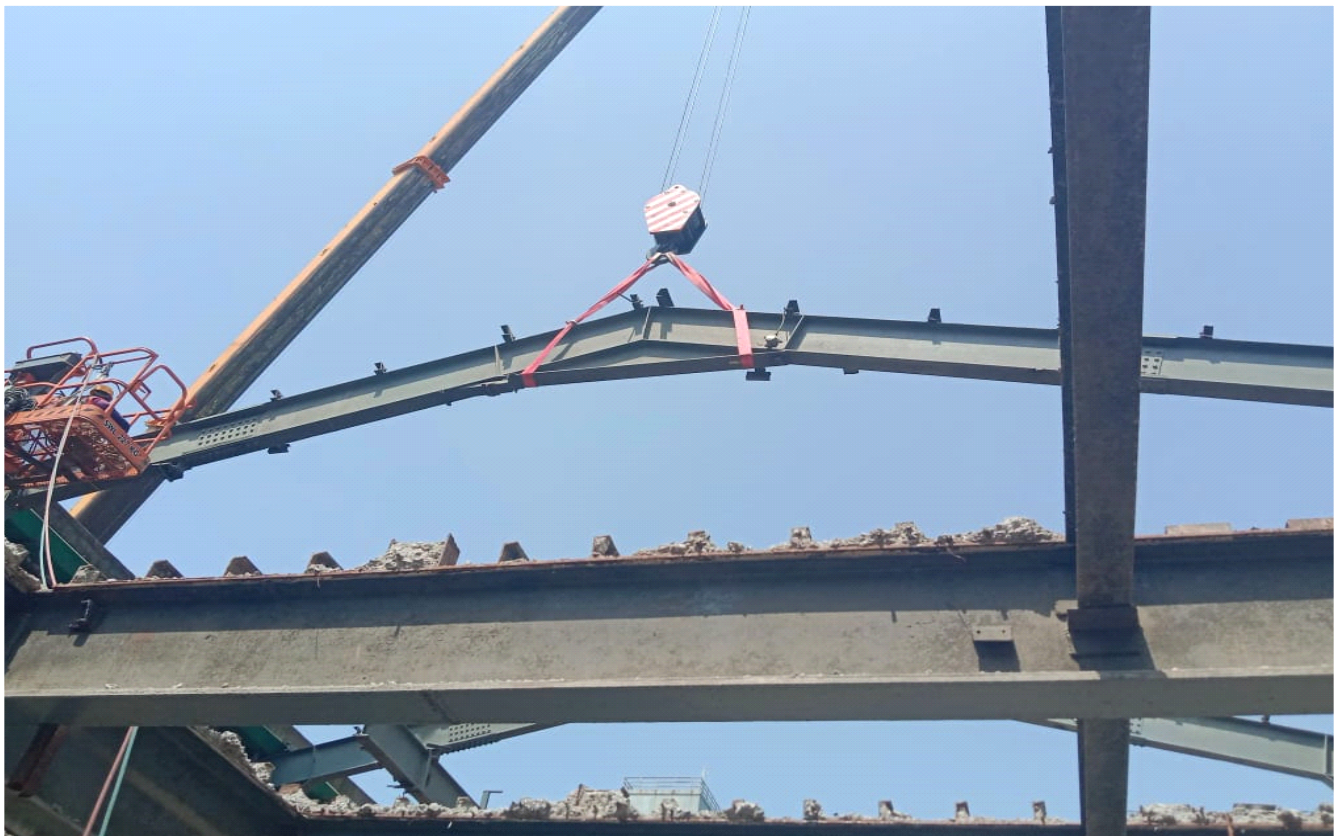
Dismantling of 15 Meter Long MS-I beam
