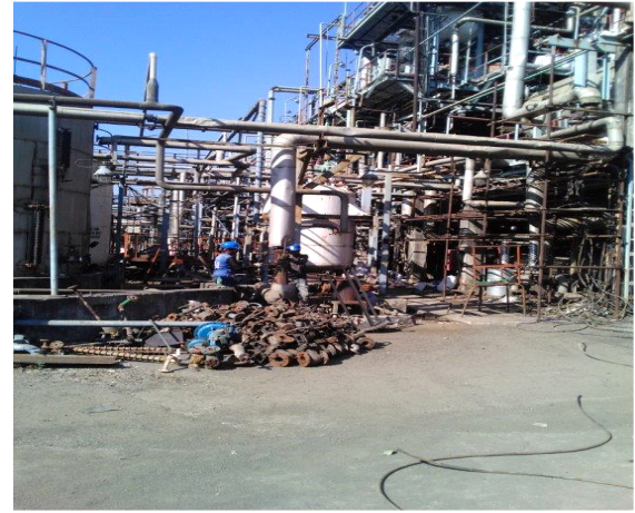
Removal of Structure column & Staircase work in progress
